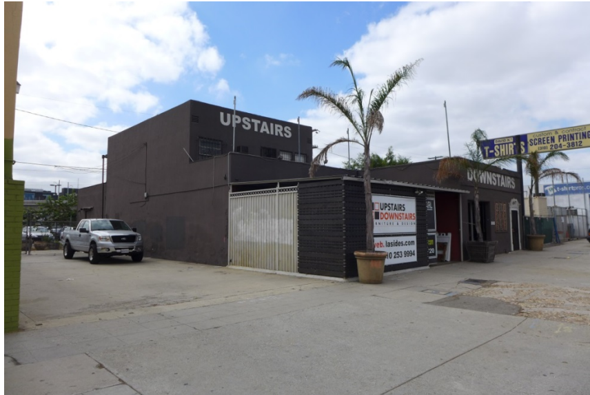
Figure 14. Primary (North) and Side (East) Elevations of 8916 Venice Boulevard, View West (PCR 2015)
