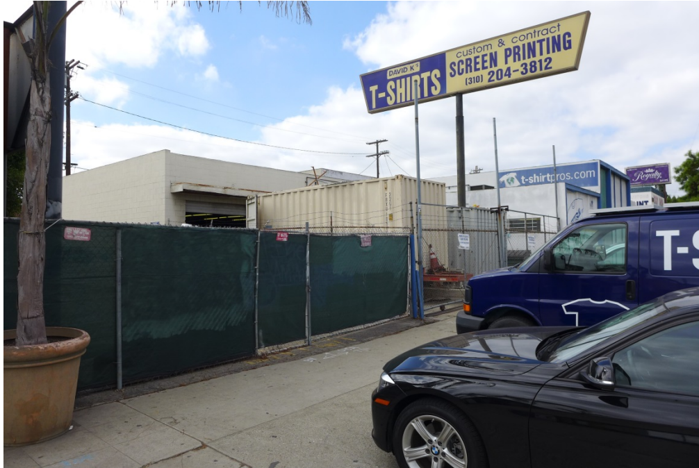
Figure 7. Additions on the East Elevation of 8926 Venice Boulevard, View West (PCR 2015)
