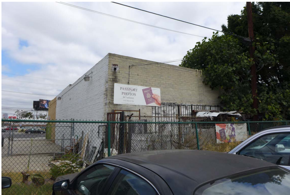
Figure 19. Rear and Side (West) Elevations of 8910 Venice Boulevard, View North (PCR 2015)
