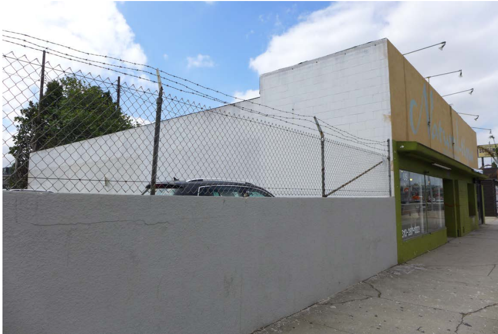
Figure 20. Primary (North) and Side (East) Elevations of 8910 Venice Boulevard, View West (PCR 2015)
