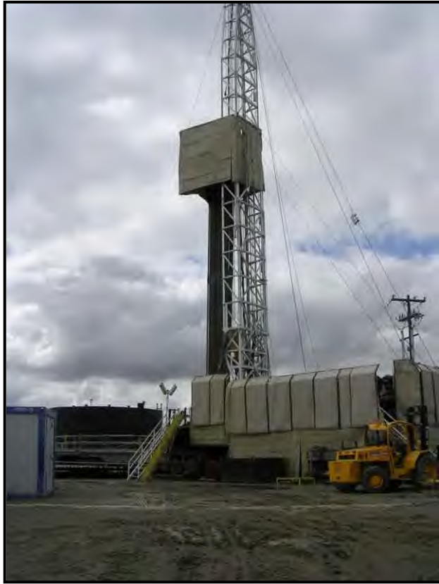
Drill rig with noise abatement pads
