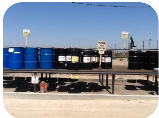
Hazardous Material Storage with Secondary Containment Curb
