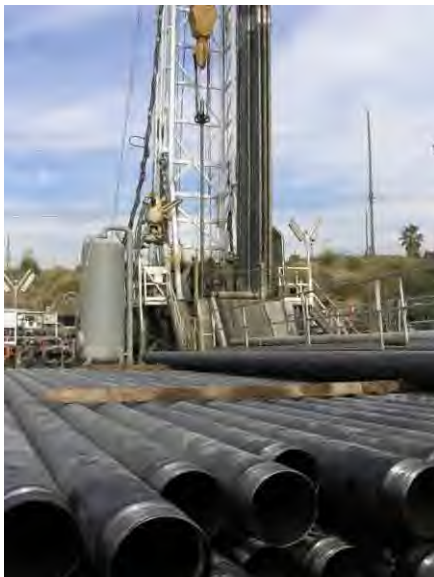
Drill Site – Production Casing Rack
