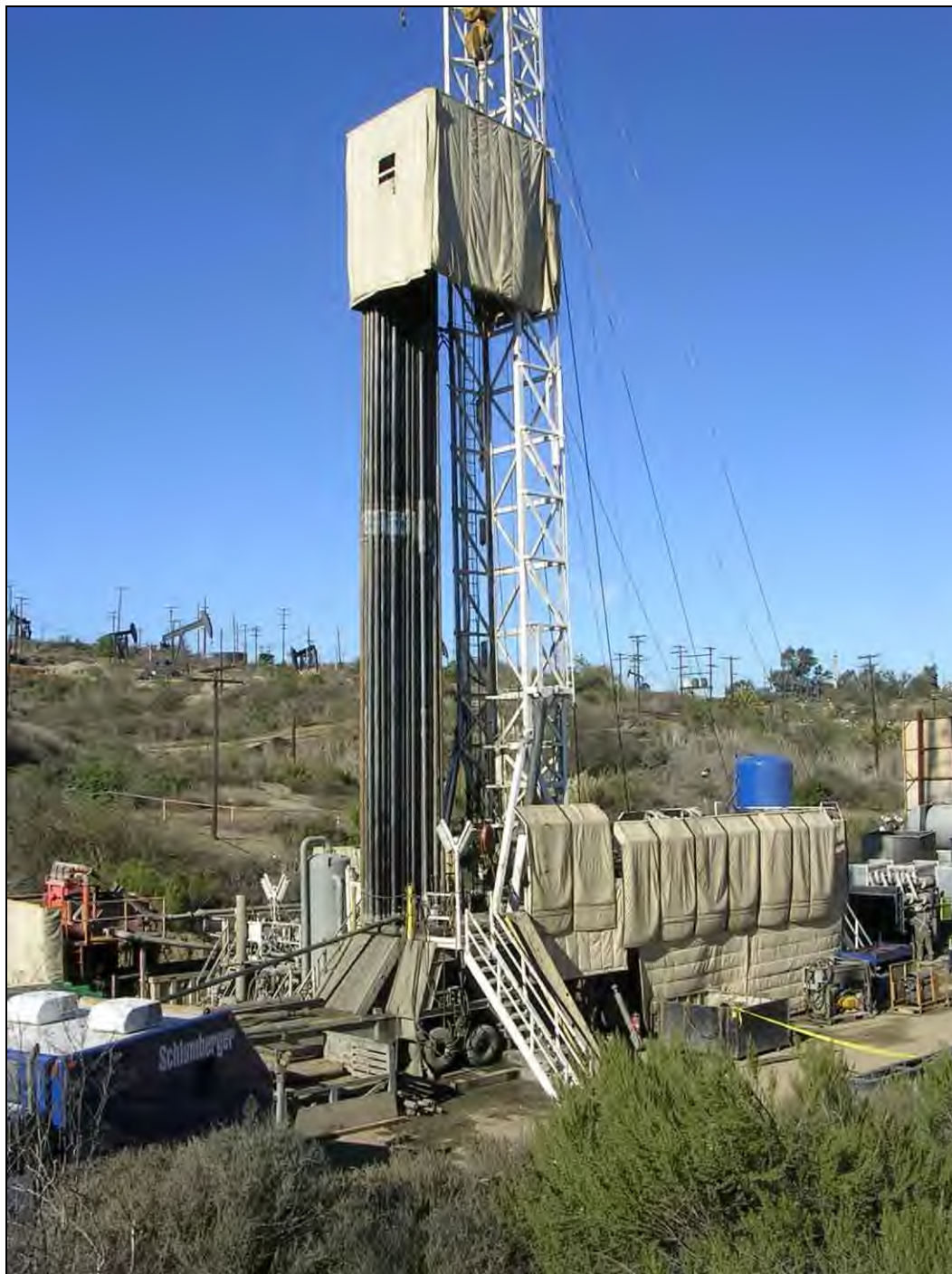
Drill Rig with Noise pads around the boards and rig floor
