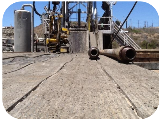
Drill Rig Pipe Rack and "V" Door Noise Dampening Rubber Surfaces
