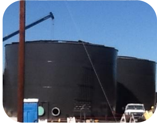
New Water Plant Tank Paint
