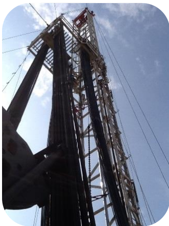
Workover Rig Derrick with Pipe
