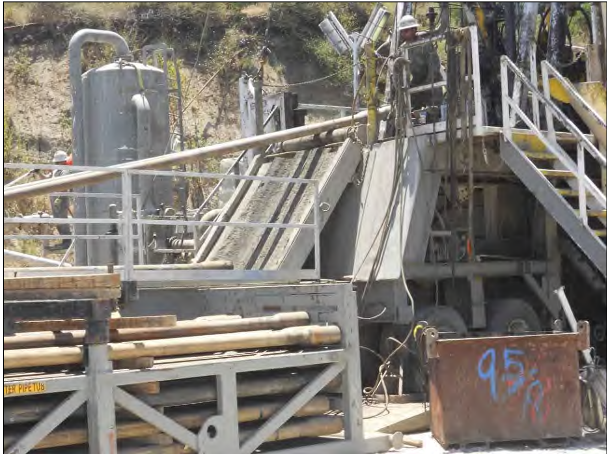
Drill Rig showing pads on V-door area and pipe lifting
