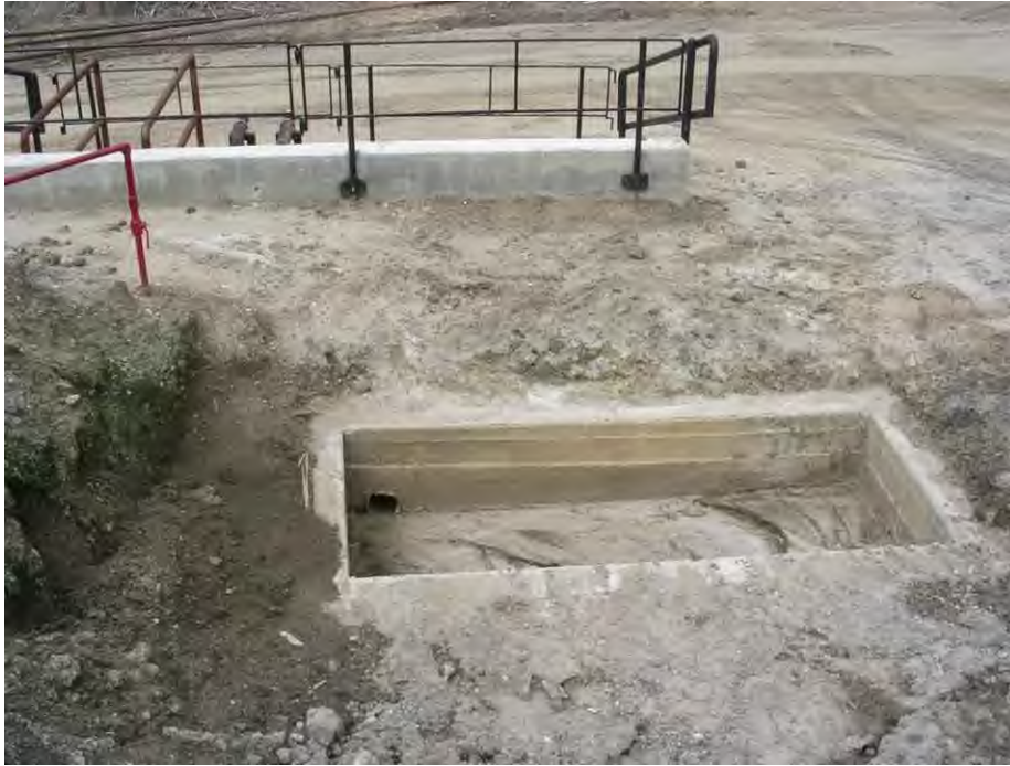
Biofarm LAI South – Culvert
