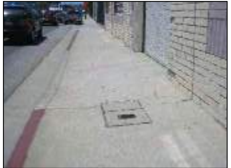
RECONSTRUCT DRIVEWAY TO MEET ADA REQUIREMENTS.
