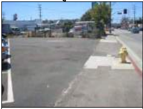
REMOVE AND RECONSTRUCT CURB, GUTTER, AND SIDEWALK AS NEEDED. OPPORTUNITY TO ACQUIRE UNUSED AREA FOR LANDSCAPING AND/OR LID FEATURES.
