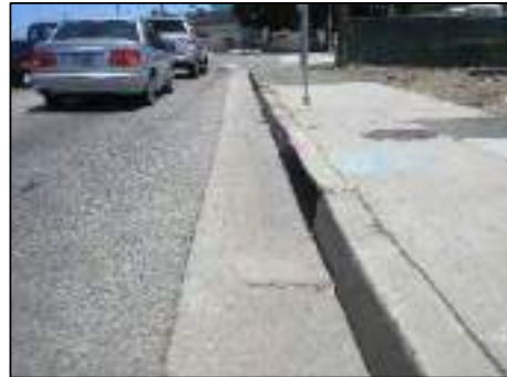
EX. CATCH BASIN. INSTALL CITY APPROVED CATCH BASIN SCREEN AND/OR DEBRIS COLLECTOR (BMP).
