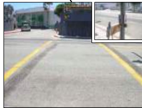
UPGRADE CROSSWALK TO CONTINENTAL CROSSWALK OR WITH DECORATIVE PAVERS. UPGRADE ALL PEDESTRIAN PUSH BUTTONS TO CITY APPROVED APS UNITS. TYPICAL FOR ALL PPB'S AT THIS LOCATION.
