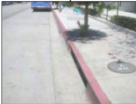
EX. CATCH BASIN. INSTALL CITY APPROVED CATCH BASIN SCREEN AND/OR DEBRIS COLLECTOR (BMP). OPPORTUNITY TO REMOVE ADJACENT TREE & REPLACE WITH STORM WATER BIORETENTION FILTRATION SYSTEM/TREE WELL (LID)
