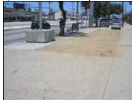
OPPORTUNITY TO CONSTRUCT BUS PULL OUT WITH CONCRETE BUS PAD. RELOCATE SIGNS AND STREET FURNITURE.
