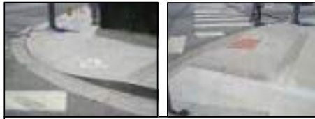
EXISTING RAMP DOES NOT MEET ADA REQUIREMENTS. RECONSTRUCT RAMP TO MEET ADA REQUIREMENTS.
