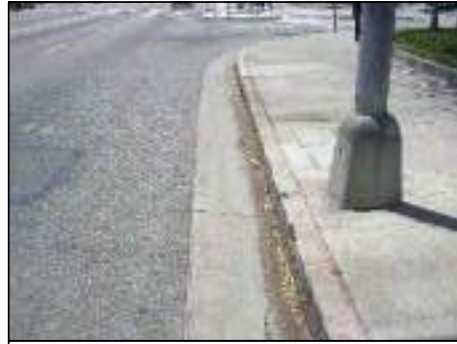
REMOVE AND REPLACE DAMAGED CURB AND CUTTER.
