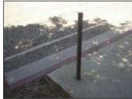
REMOVE ALL REMAINING UNUSED PARKING METER POLES (TYPICAL).
