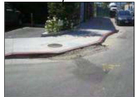
EX./RECONSTRUCTED CATCH BASIN. INSTALL CITY APPROVED CATCH BASIN SCREEN AND/OR DEBRIS COLLECTOR (BMP).
