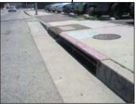
EX. CATCH BASIN. INSTALL CITY APPROVED CATCH BASIN SCREEN AND/OR DEBRIS COLLECTOR (BMP).
