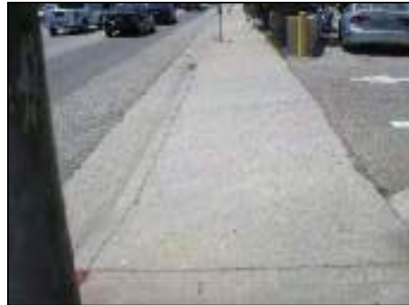
RECONSTRUCT DRIVEWAYS TO MEET ADA REQUIREMENTS.
