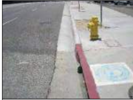
VACANT TREE WELLS. OPPORTUNITY FOR MULTIPLE BIO-RETENTION FILTRATION PLANTERS (LID) AND CONNECTION TO ADJACENT CATCH BASIN.
