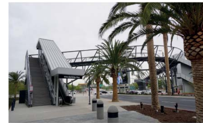
Pedestrian Bridge Example
