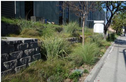
City Maintenance Operations Building location: landscape in front of a building Collects rain water from roof
