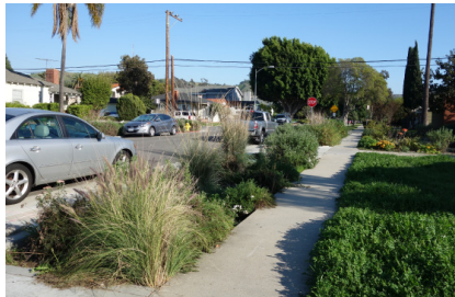
Baldwin Ave. and Farragut Dr. location: parkway Collects rain water from street
