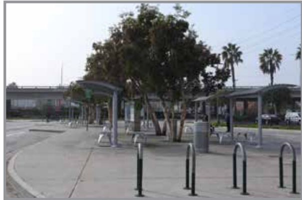
Westfield Culver City Transit Center
