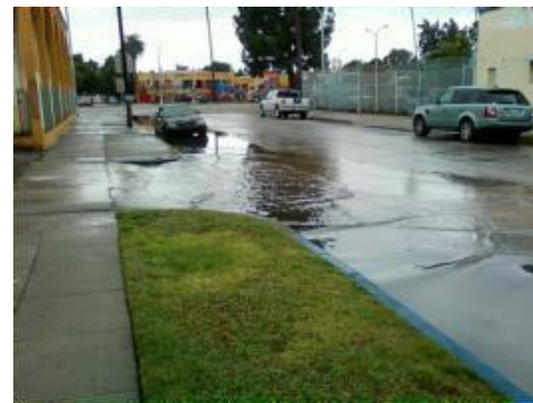
Figure 5-14 Existing Wet-Weather Flooding and Ponding Along the Proposed Vermont Avenue Project Site
