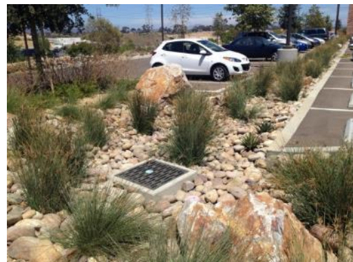
Figure 5-11 Recently Constructed Biofiltration in a Parking Lot
